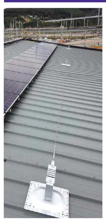
The **KEELINE** horizontal lifeline system is designed to provide safe access to any area of a roof by allowing workers to be permanently attached to the line at all times and be able to freely move around the roof surface. The system utilises 8mm grade 316 stainless steel wire and allow spans of up to 12m between posts and can be utilised by up to three users at any one time.
