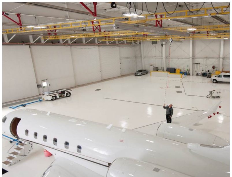
Figure 1- Traveling Bridge Fall Protection System
